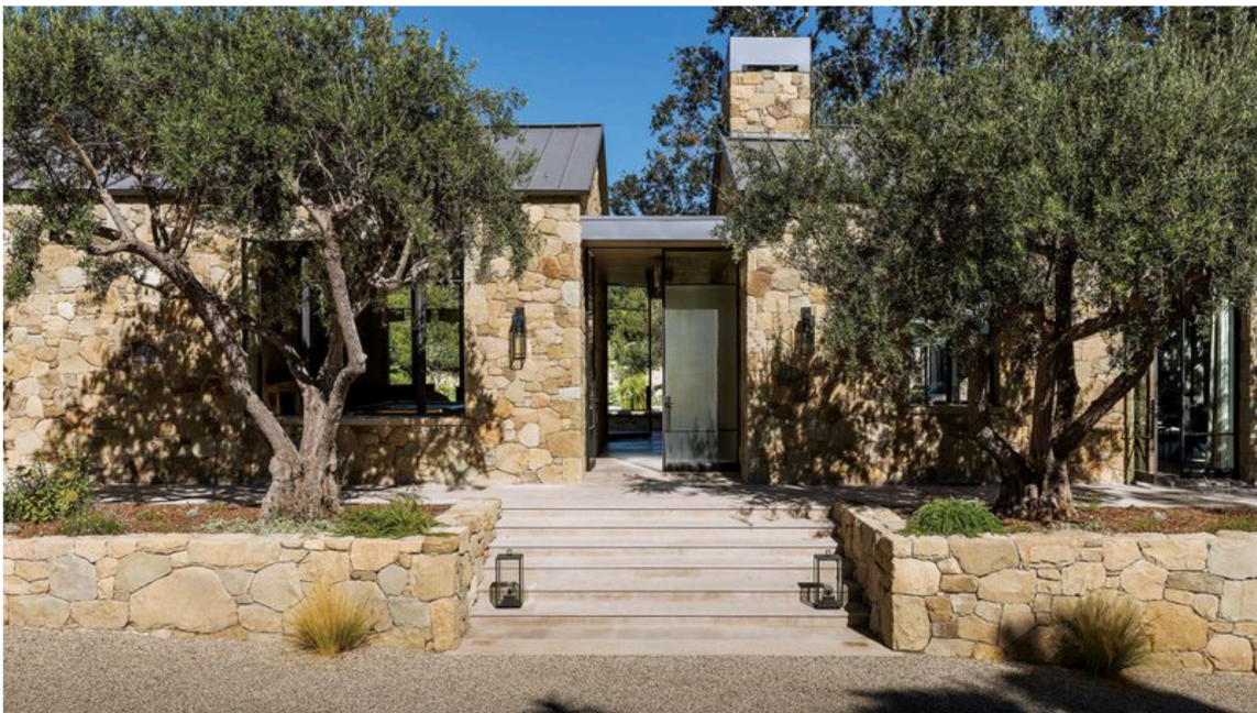
Metal roofs, steel window and door frames, and stone quarried from the site define William Hefner and Kazuko Hoshino's family retreat. (Richard Powers)
